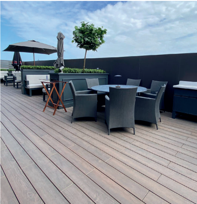
PRIVATE ROOF TERRACE · CORNWALL · EXADECK TECA
