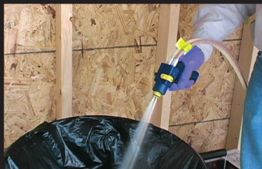
Calibrate foam in waste container.
