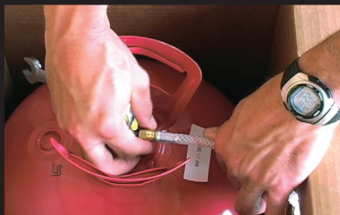
Attach color coded hoses.
