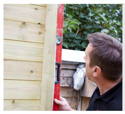
**Tip:** If the panels are not plumb or one is slightly higher than the other plastic packers can be slid under the wall panel to raise them slightly to get them level. The reason for this will be down to tolerances in the base and/or panels etc. The panels do not need to be perfectly level at the top as this is all covered by the roof. It is more important that they are plumb.
