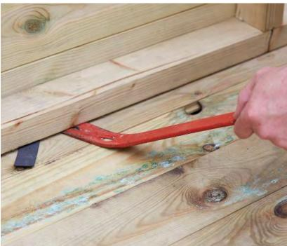
Continue to fit the remainder of the walls in the same way ensure the panels are in the correct position and fully pulled up against the base (floor). When installing the panels that butt together coach bolts and washers are provided so these can be used to hold them together through the pre-drilled holes.
