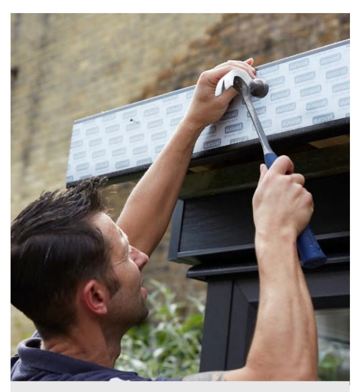
Fit the larger fascia boards to the roof as shown below using the poly pins provided. The top of the fascia board should align with the top of the roof at this stage.
